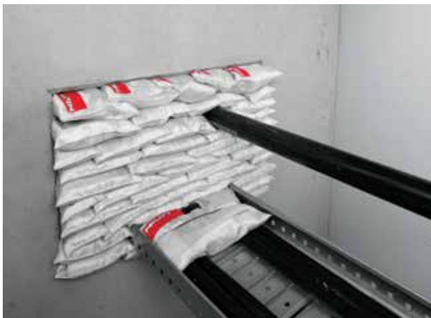
Penetration gap protected with intumescent bags. (Source: Hilti)
