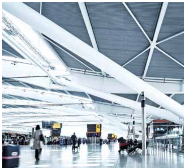
Example of a reactive (intumescent) coating of a structural steel element at Heathrow
